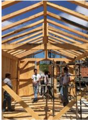
Image 33 - Is the shelter a solid structure?
