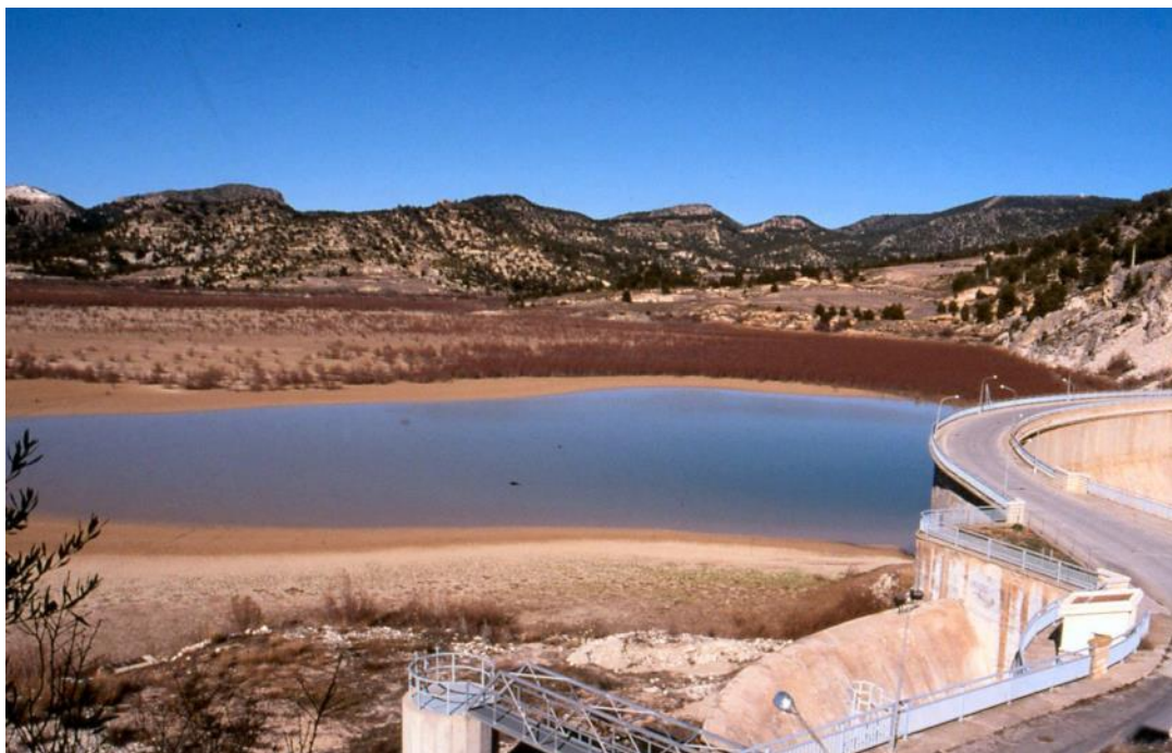
Image 6 - View of the Valdeinfierno reservoir (south-eastern Spain) that lost most of its storage capacity due to soil erosion and siltation (© J. de Vente).
