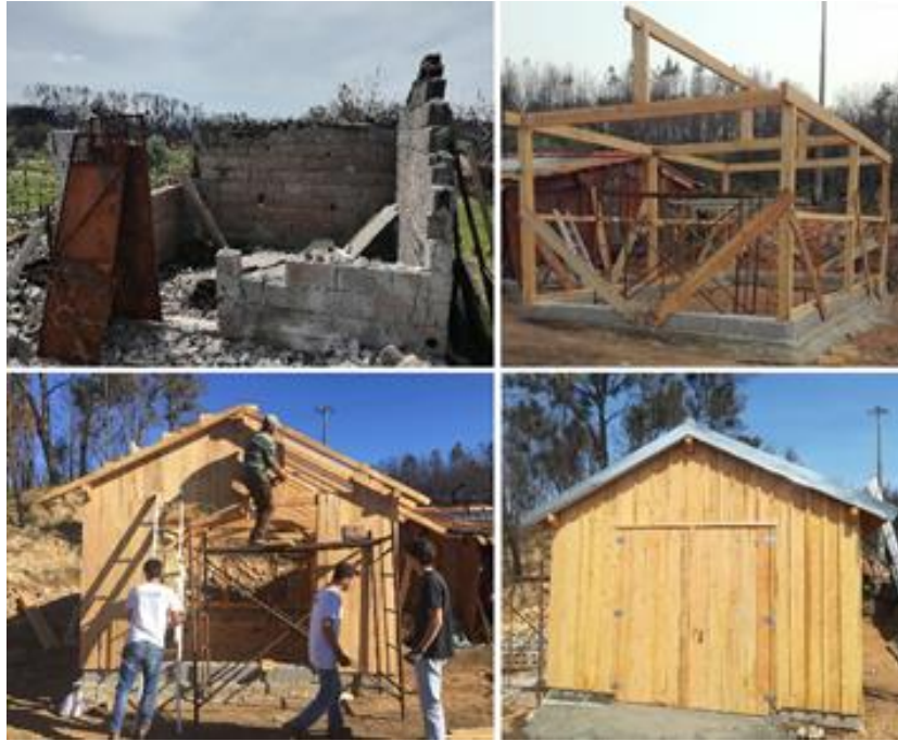
Image 9 - The construction of a new shelter
